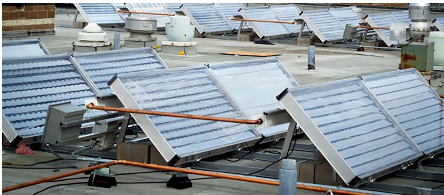
The new solar thermal system is expected to annually reduce the Guterman facility’s campus steam consumption by 122 million Btus and offset approximately 4% of the facility’s summer heat load. (Lindsay France/Cornell University)
